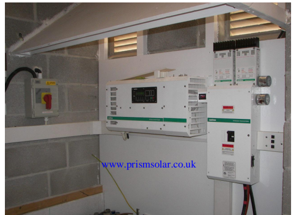
Here you can see my original 2x C40 (PWM) charge controllers each handling 1200 watts of PV Panels each
