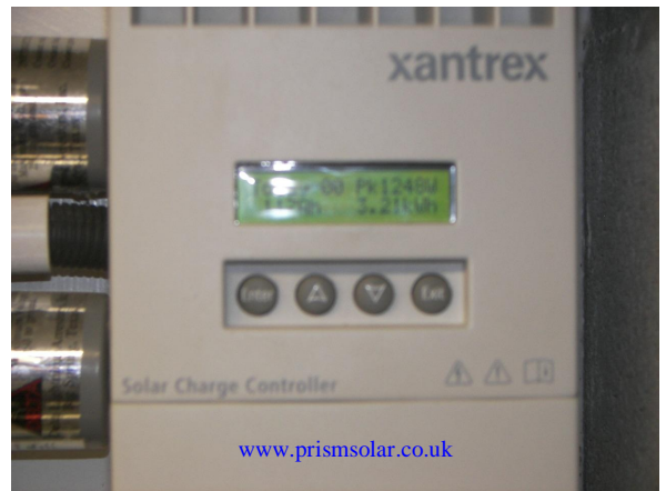
If you look closely at the top right-hand corner of the LCD display you can see a PK1248W . That was a one day peak recording of 1280 watts being sent to my batteries .Which considering my array is rated 1200 w STC is proof of the Electronic Magic that MPPT offers . I have seen a recorded peak of 1440 watts, honestly !
