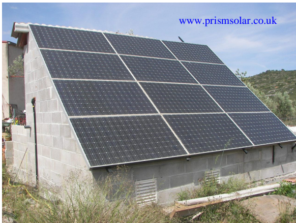
12 x 200w Mono Panels (2400w) wired all in parallel to 2 Xantrex C40 PWM Charge Controllers (24v nominal)
